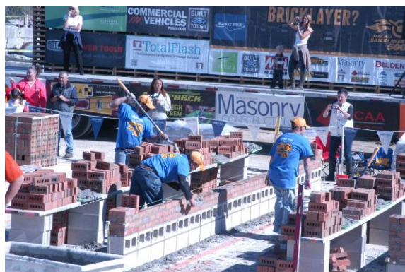
Masons in Action
